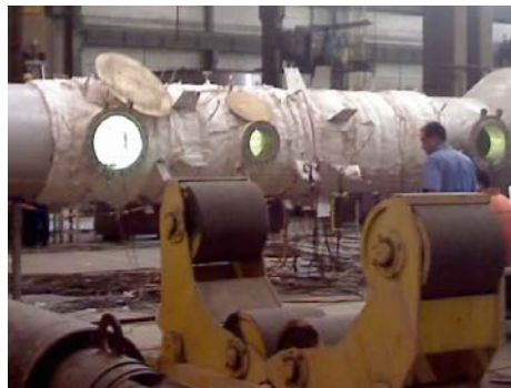
Curing with the help of wrapped heating elements
