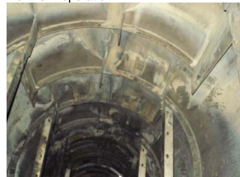
Inner tower wall after repair elements
