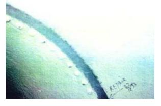
Coating of the inner respectively outer diameter of a penstock pipe with diameter appr. 1,5 m, length appr. 900 m. Damages were caused by erosion and abrasion due to water and sand. The coating was affected with Ceramium pasty with Hardener CE.
