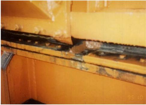
A leakage on a transformer (240.000 kVA) was repaired with MM-metal oL-steelceramic and Hardener red without cutting of the station. After this a second layer with MM-metal oL-steelceramic and Hardener yellow was applied.
